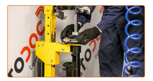
Install the rubber spring spacer.
