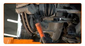
Install a new arm. Use a rubber mallet. Use a crowbar.
