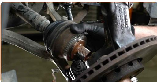
Replacement: CV joint – VW PASSAT Variant (3B5). Tip from AUTODOC experts:
