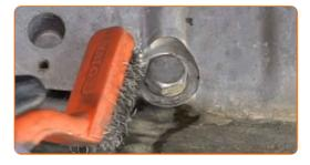
Unscrew the drain plug. Use a drive socket #19. Use a ratchet wrench.
