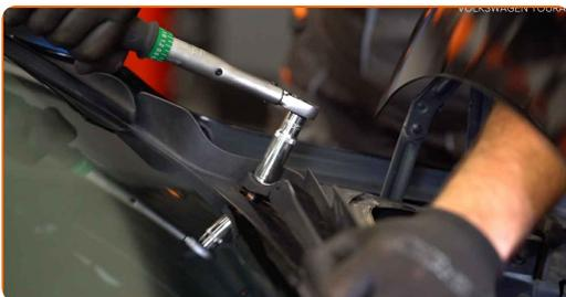
Replacement: suspension strut – VW Beetle Convertible (5C7, 5C8).
