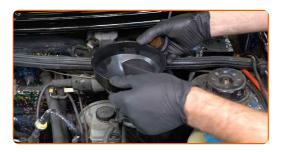
Pour coolant in the coolant reservoir.
