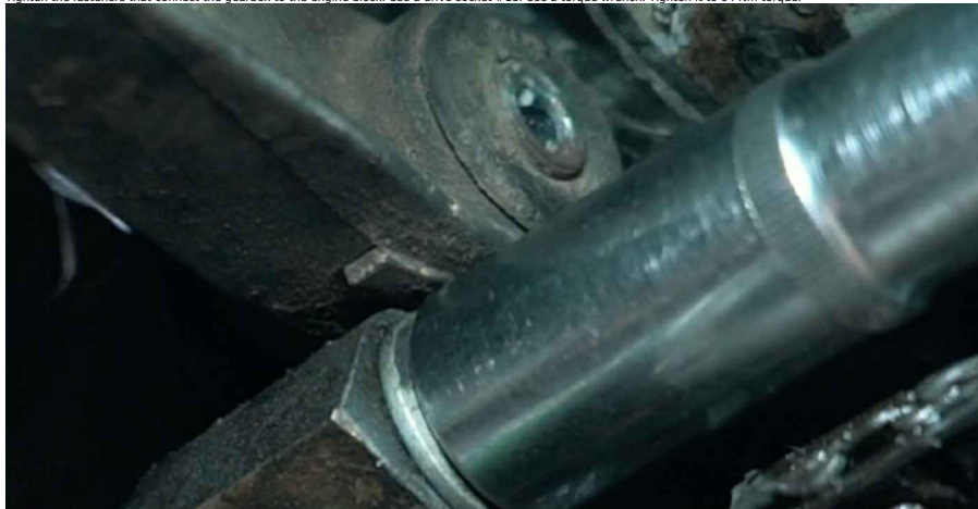
69 Install the lower gearbox mount.
