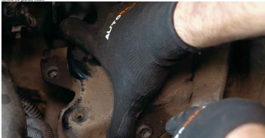
club.autodoc.co.uk 12-32 45 Unscrew the fasteners that connect the bottom gearbox mount to the gearbox. Use a combination spanner #16.
