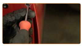
Remove the cover from the exterior door handle fastener. Use a plastic trim tool.
