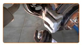
Unscrew the brake caliper fastening. Use a drive socket #14. Use a tap wrench.
