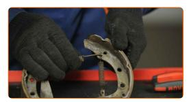
Remove both shoes from the mounting bracket. Use round-nose pliers.
