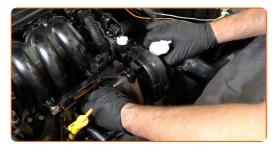
Screw in the fasteners connecting the secondary air pump to its bracket. Use a combination spanner #10.
