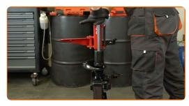
60 Install a spring on the strut.
