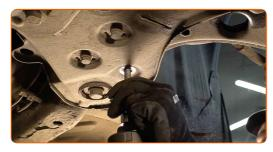
Release the fastener connecting the ball joint to the steering knuckle. Use a crowbar. Use a hammer.
