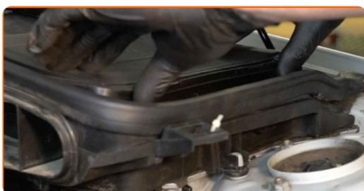
**50** Install the air duct housing.
