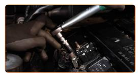
Treat the ignition coil connector with electronic spray. Use dielectric grease.
